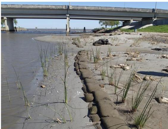
**Close-up of the retaining wall filled with dredge material and newly planted marsh grass**
